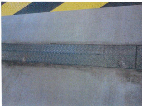
Renforcement joint de dilatation
